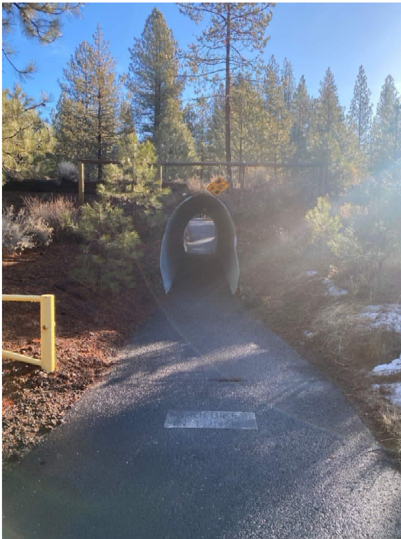
West Approach to Tunnel
