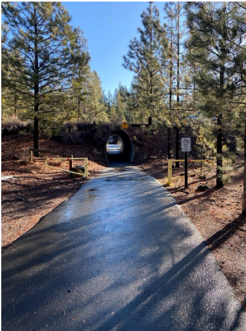
West Approach to Tunnel
