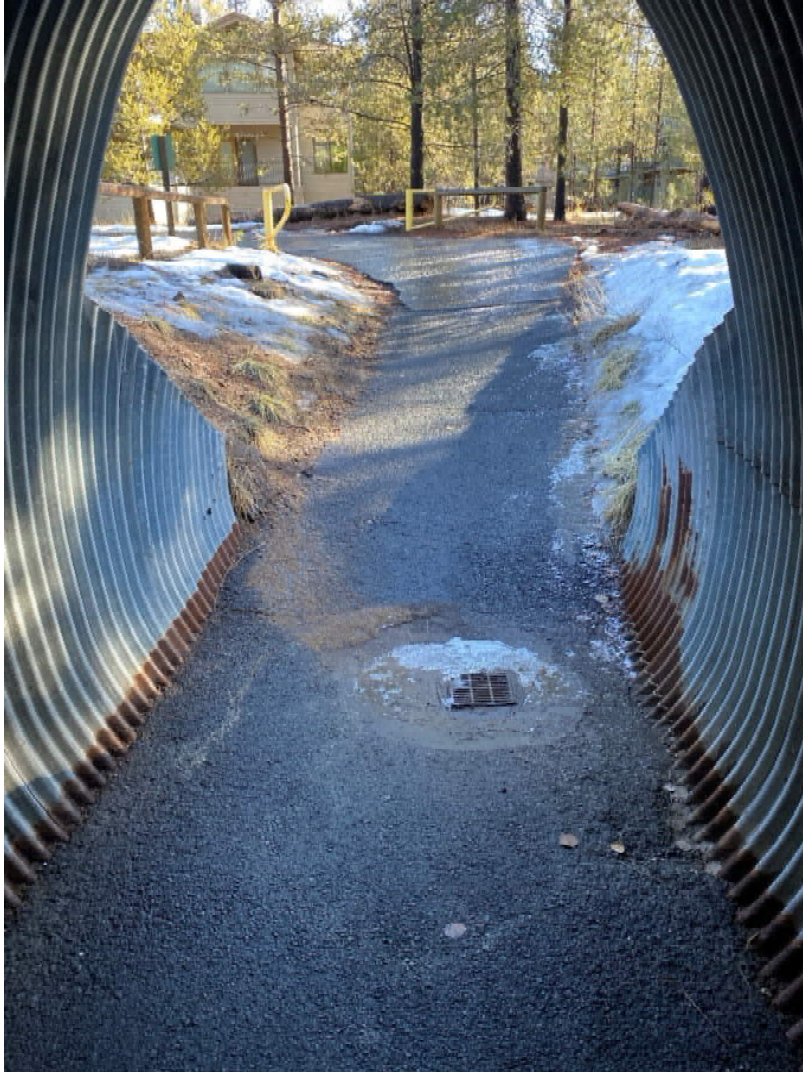
Existing Area Drain
