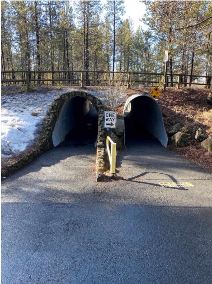
North Approach to Tunnels
