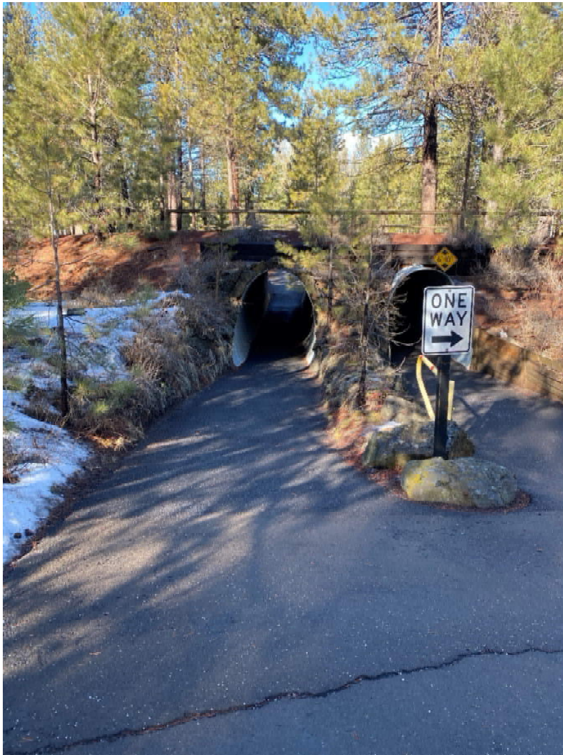
East Approach to Tunnel
