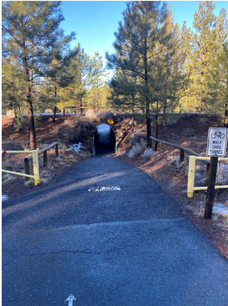
East Approach to Tunnel
