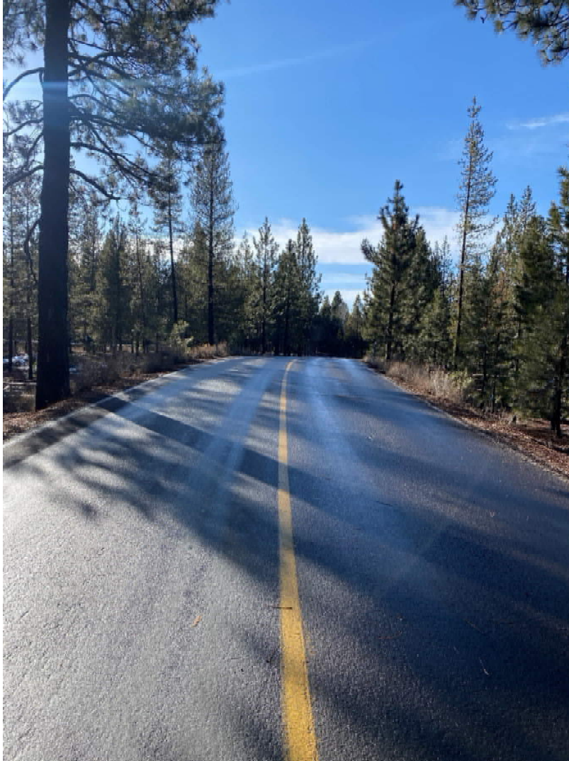
Theater Drive crossing over tunnel
