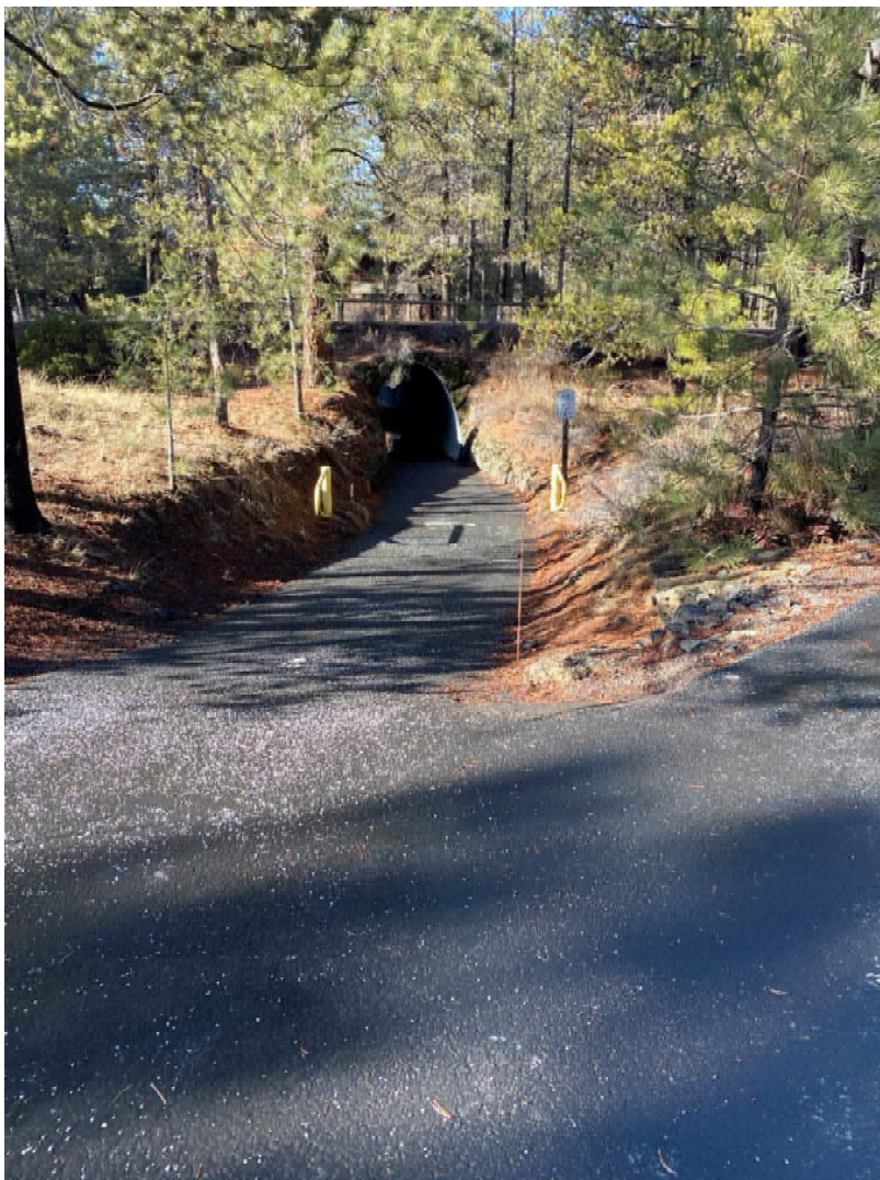
East Approach to Tunnel
