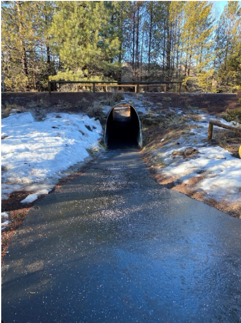
East Approach to Tunnel
