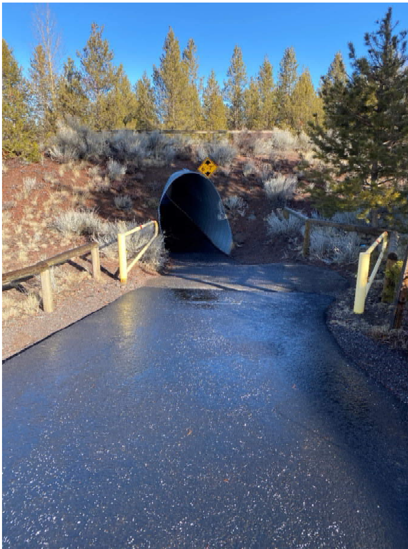
South Approach to Tunnel
