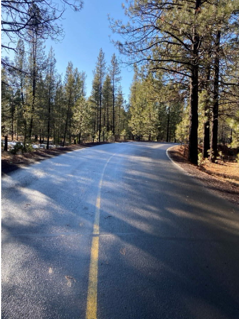
Abbot Drive crossing Tunnels from North
