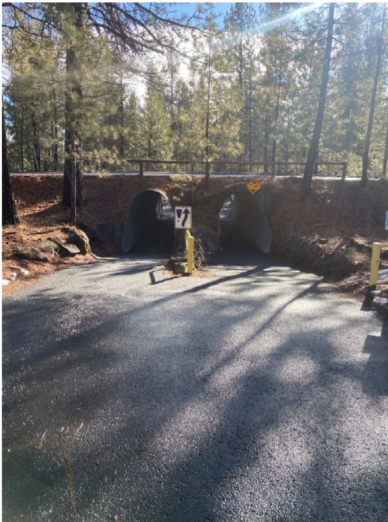
West Approach to Tunnel
