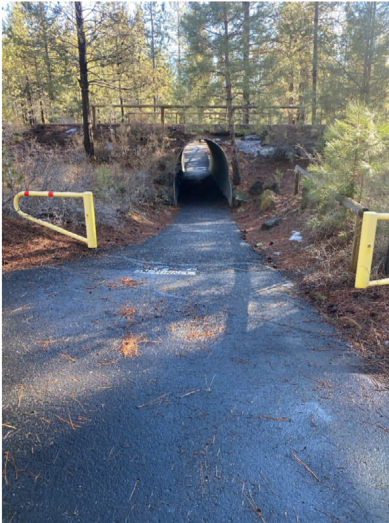
West Approach to Tunnel
