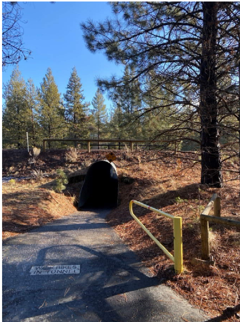
West Approach to Tunnel
