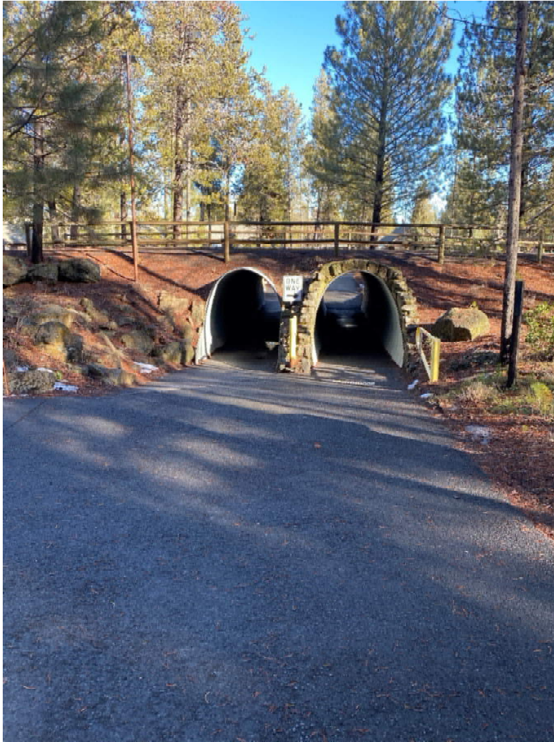
South Approach to Tunnels
