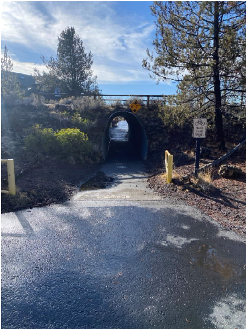
North Approach to Tunnel
