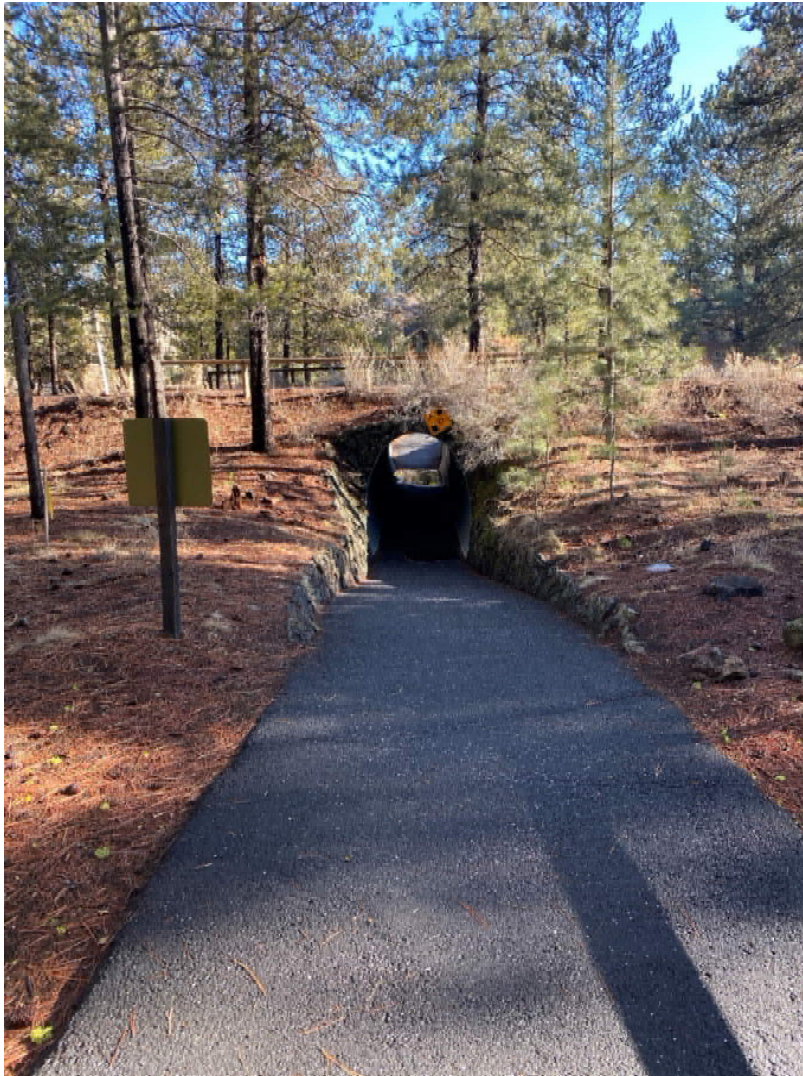
West Approach to Tunnel
