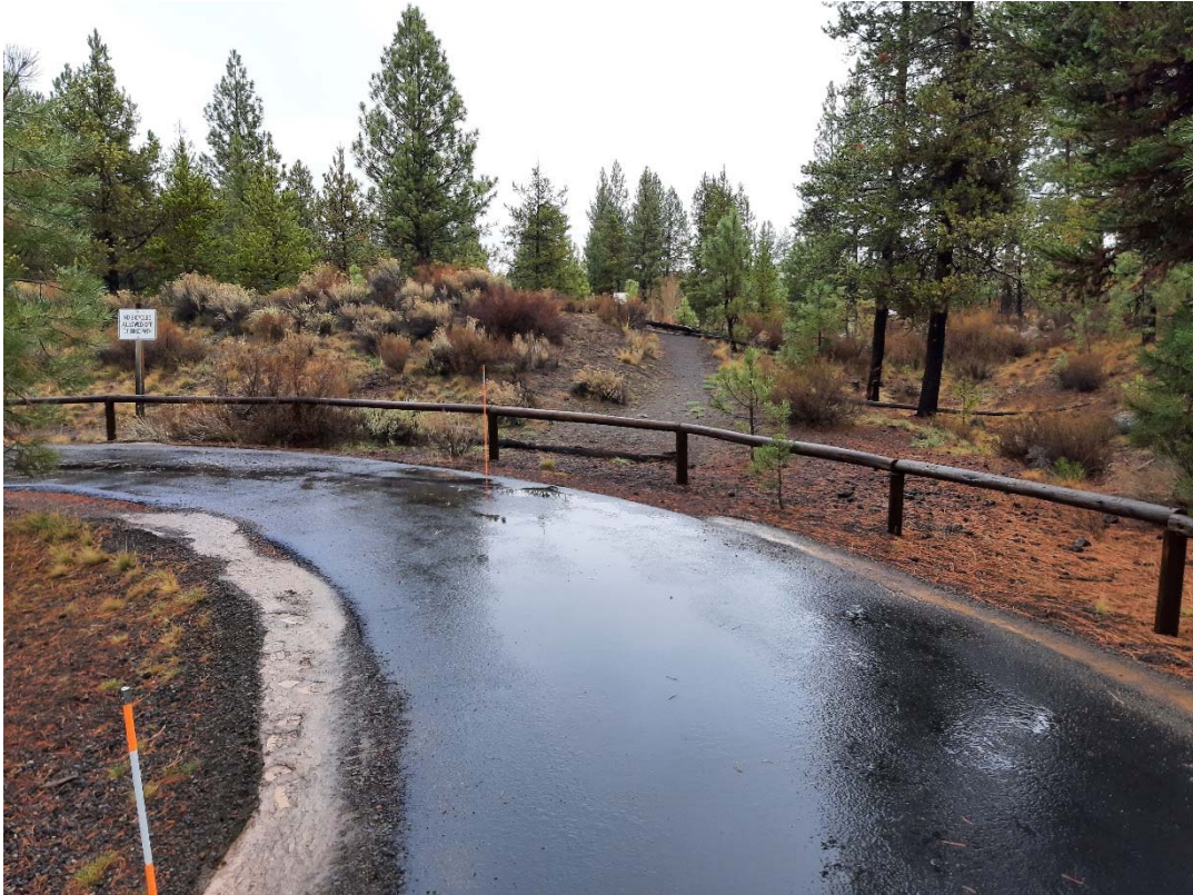
Facing Approximate Proposed Tunnel Location from South Side of Theater
