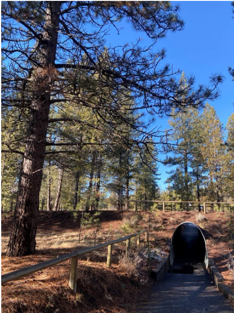
East Approach to Tunnel
