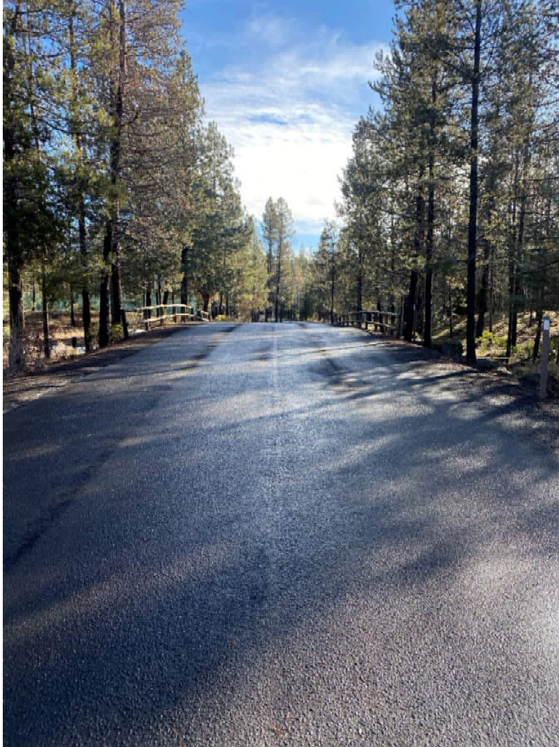
Center Drive over Tunnels with Surrounding Trees
