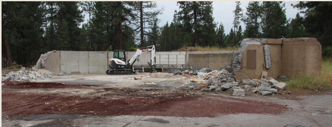
Public Works Old Roundhouse Demolition
